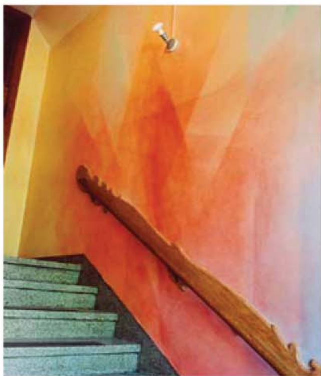
Lazure "rainbow" treatment of a stairway wall,
